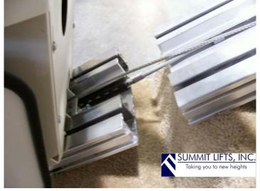
7) Use the handcrank to manually tighten the steel cable and release the Slack Cable Brake.
