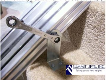
6) Slide the top piece of track uphill leaving approximately a 2" gap. Re-tighten the
