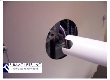
8) Without anyone sitting in the seat, carefully run the lift up until the upper set of wheels are in the gap between the tracks. (The block of wood was only used for photographic purposes and is not needed)
