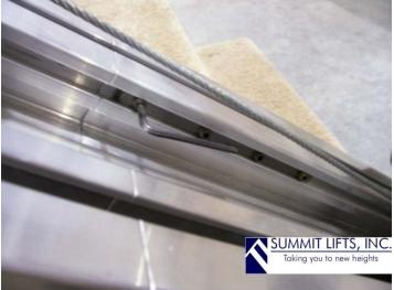
5) Loosen the track mounting brackets from the sides of the top piece of track.
